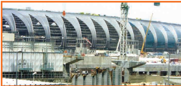
Expansion project - Dubai Airport, UAE
