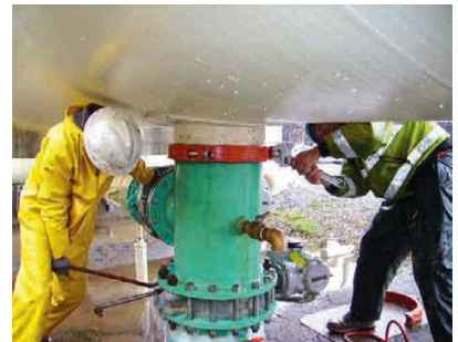
Water Treatment, USA
